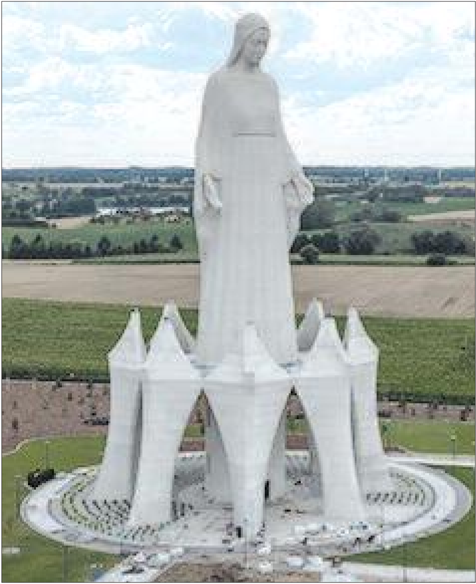
A statue of the Virgin Mary during finishing works at the construction site in Konotopie village, next to Torun, central Poland.
