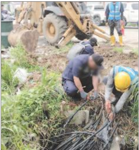
The concealed water source uncovered.
